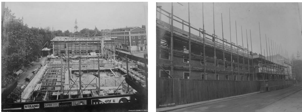
Figure 5: Left, a photo of June 1925 showing the foundations: right, a photo of October 1925 showing Drayton House and the meeting house block under construction (Friends House Library, Lidbetter Collection)
